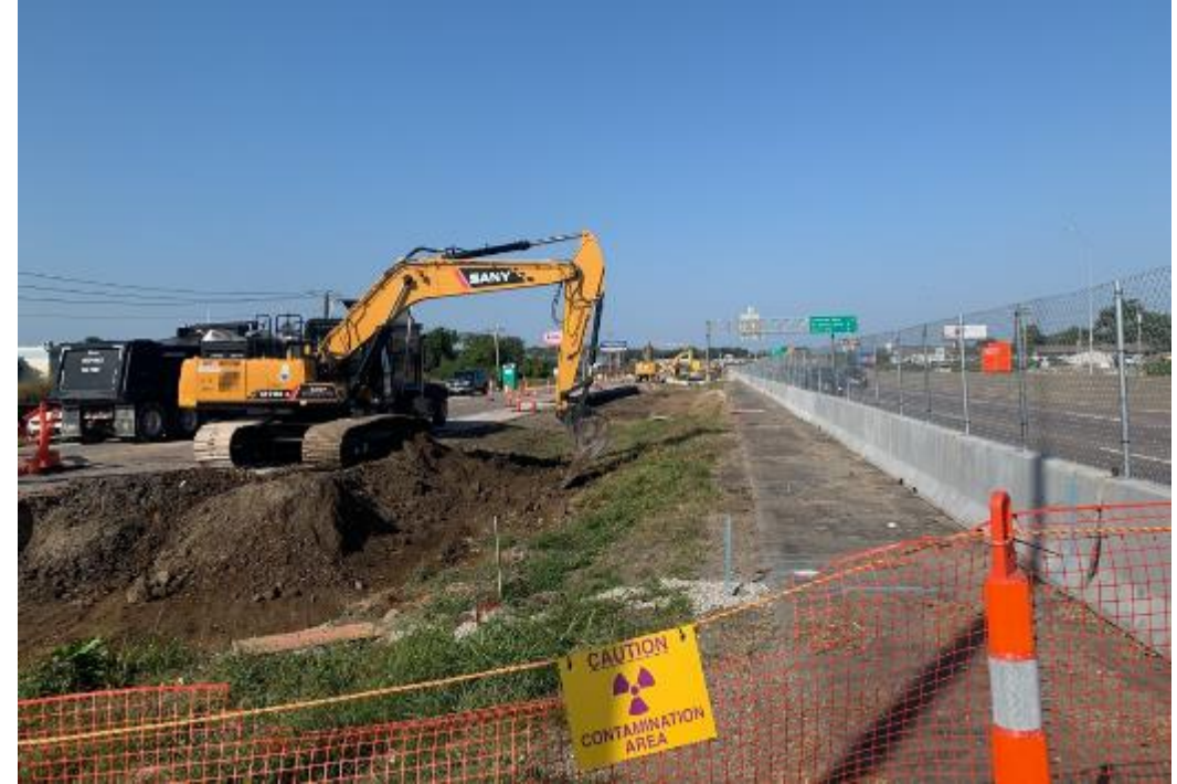
Remedial activities at Pershall Road adjacent to I-270 East Bound Lanes
