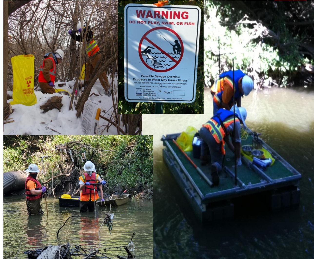
CWC sampling continues all year under all weather conditions. A special platform was built to take sediment samples in deep water.
